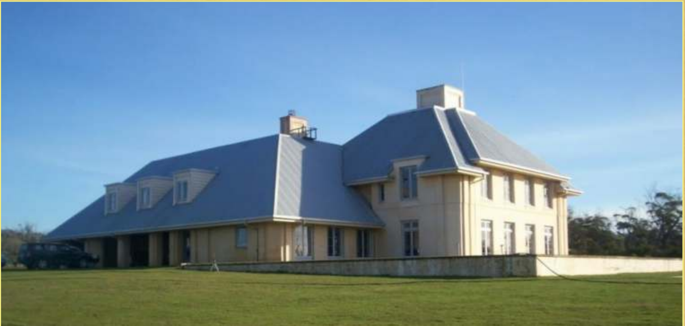
The mansion as it looked in 2007, before it was abandoned – RM
