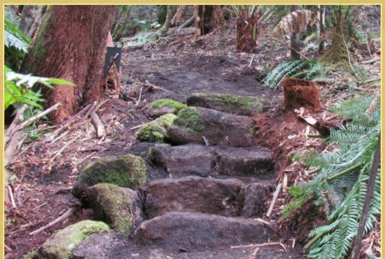
Halls Falls Track Work
