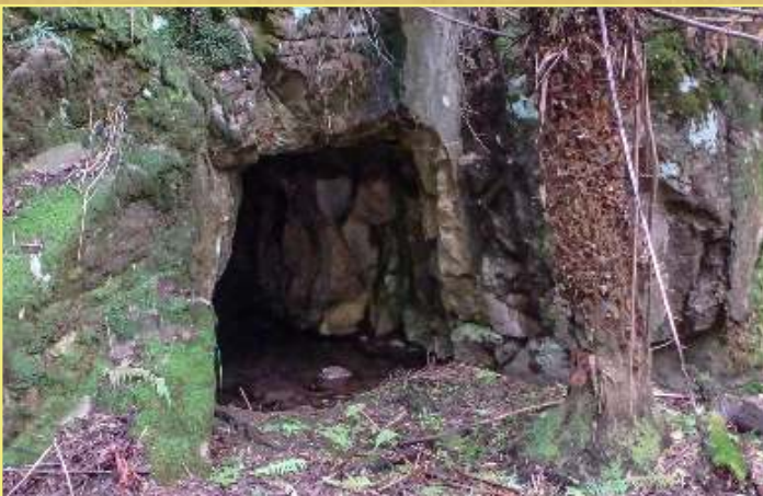
Second Derby Tunnel (RM)
