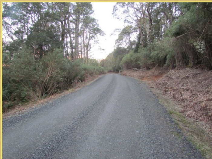
... and after restoration
