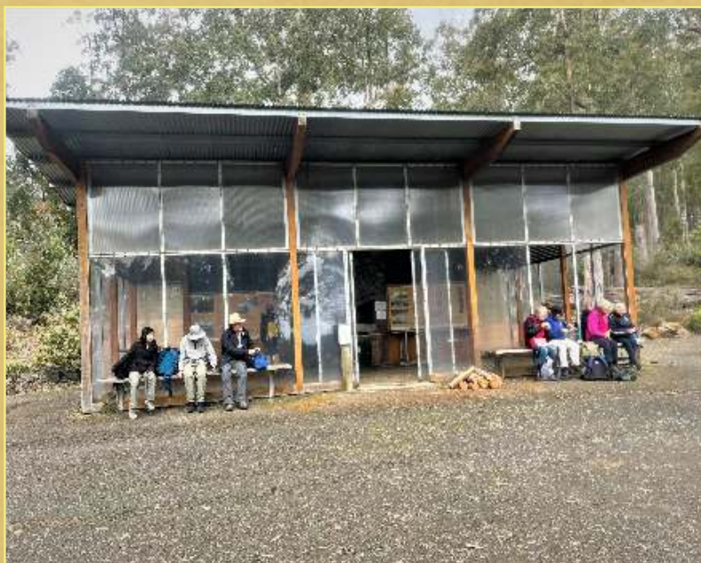
Mt Barrow Discovery Centre, completed in 2004 – CFE
