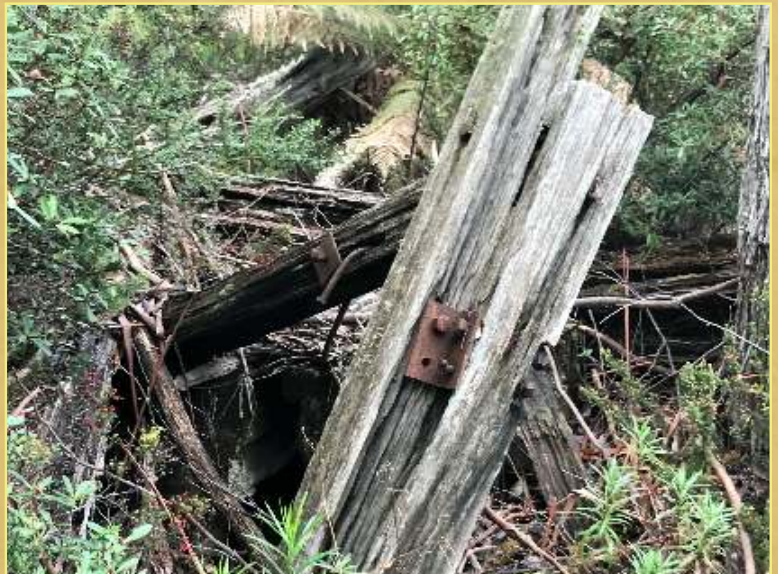
Wooden, iron, and concrete structures that were part of the old Mt Barrow sawmill – L&G A
