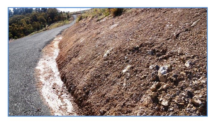
**Plate 10.** Extensive cutting exposing mudstone material.
